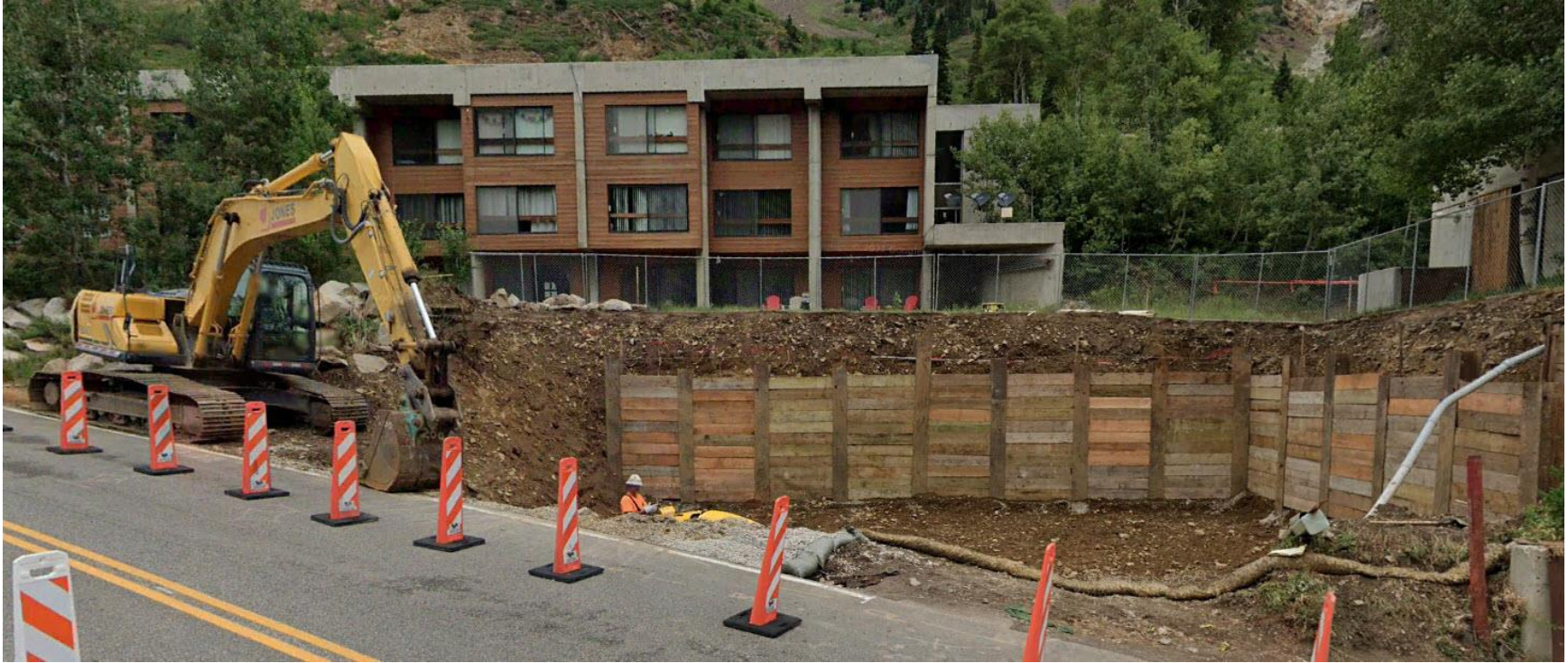
Figure 1: View of the excavation and shoring for Building 3
