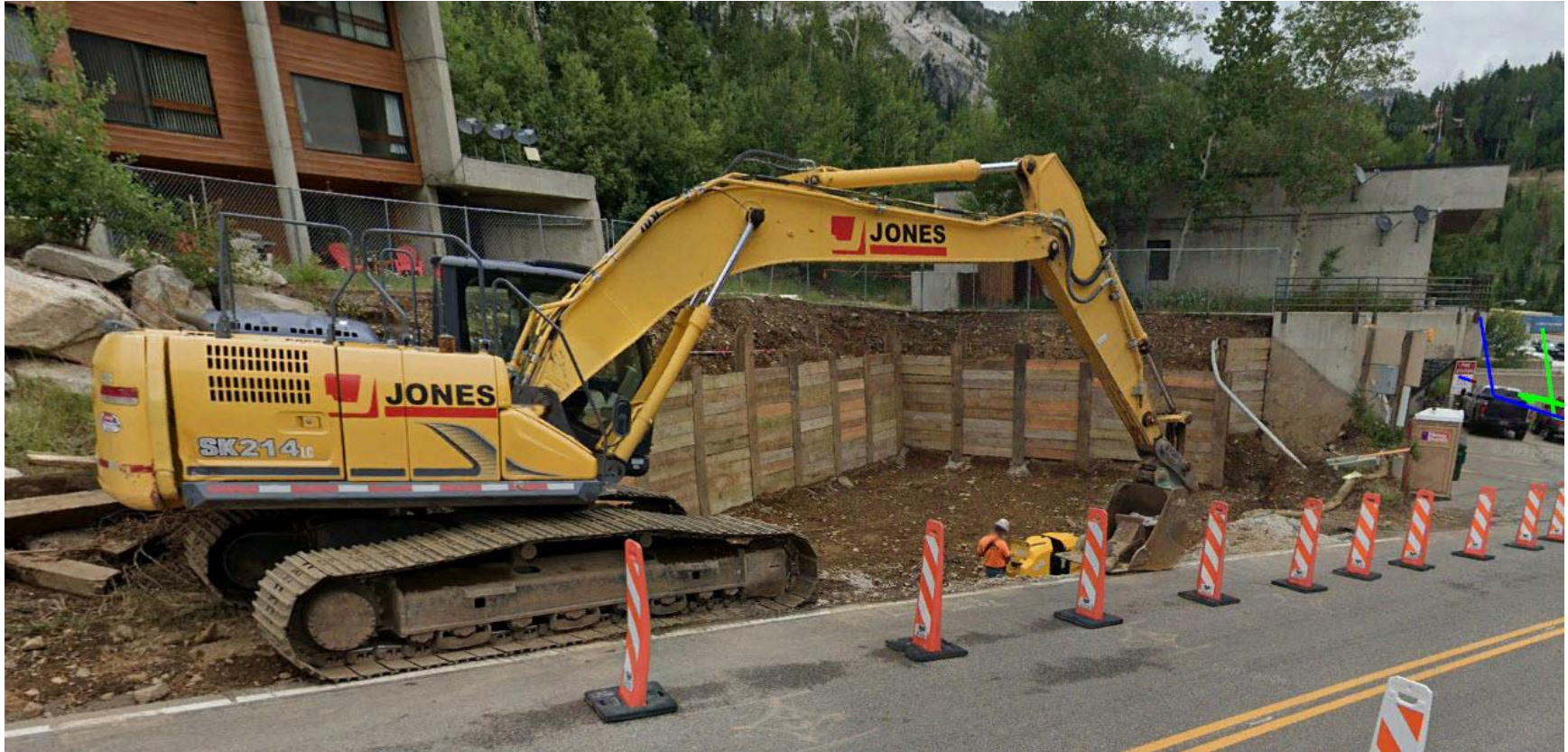
Figure 2: View of the excavation and shoring for Building 3 against the Firehouse
