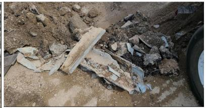
Thrust block encased an 8ft+ area of pipe encasing a large portion of the line with concrete makes the line far more brittle and susceptible to break when any additional utility is to be installed in the area See photo below of specifications of Udot roads and what was installed: Additional pictures and videos are available
