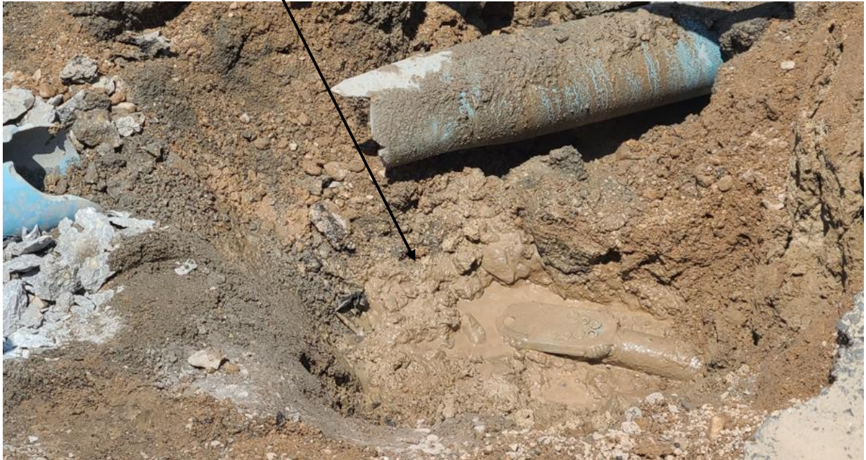
Image of large piece of asphalt in the same location, the drill head was pushing.
