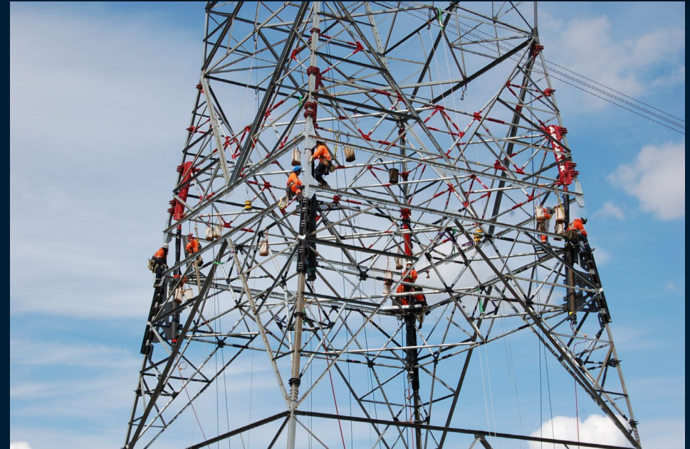
Workers raising 735 kV Tower with lines in place
