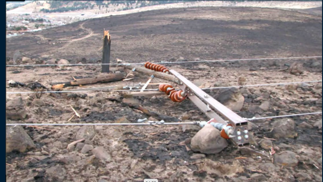
Wildfire burned the poles to the ground but HPC stayed intact
