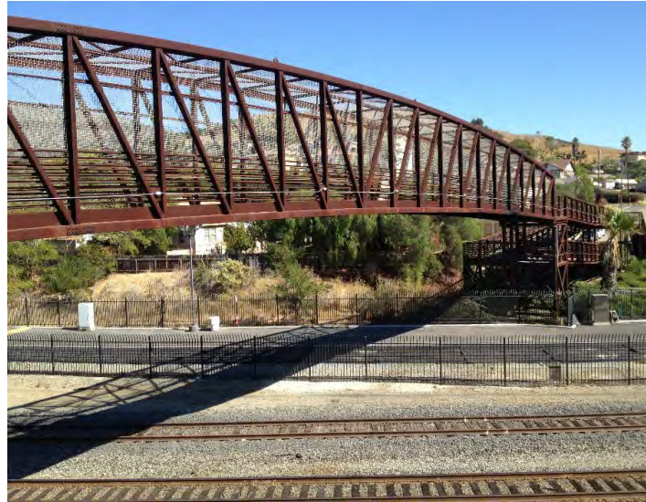
Photo: San Obispo Parkway over UP
